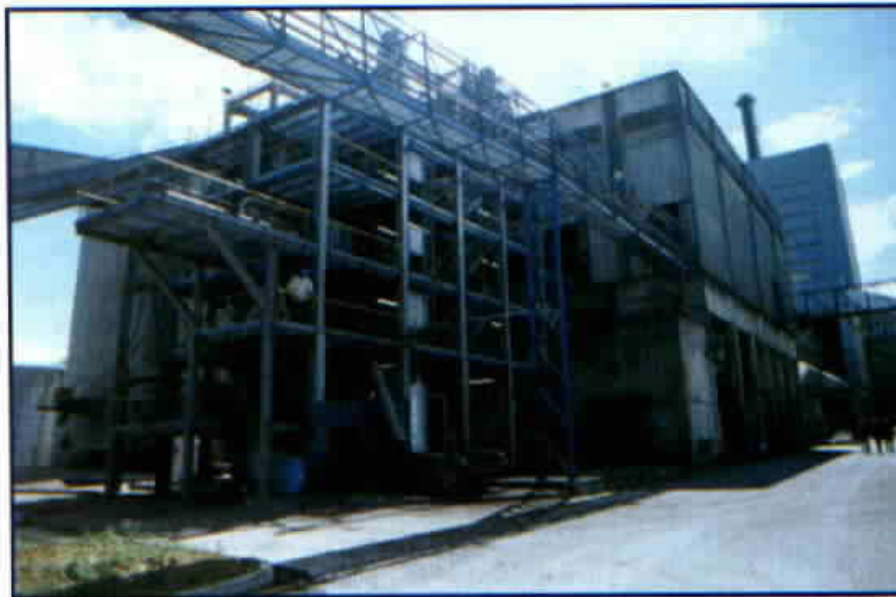
Left: The Pyrolysis unit at Rochefort-sur-Nenon, designed and built by Nesa of Belgium. Behind it is seen the main building, with cladding designed by the architect Thierry Bogaert. Computer simulations helped to guide the choice of colours, designed to blend the building into the sky.
