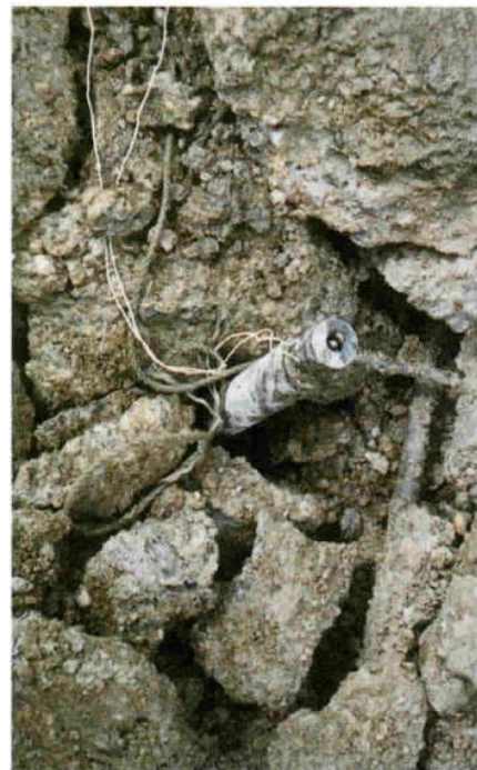
▲ Cardox at work, the rebar is separated from the fractured concrete...
