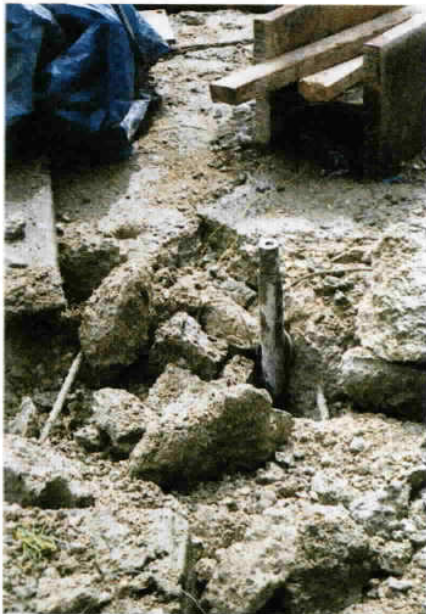
▲ ...and the Cardox tubes can be re-used
